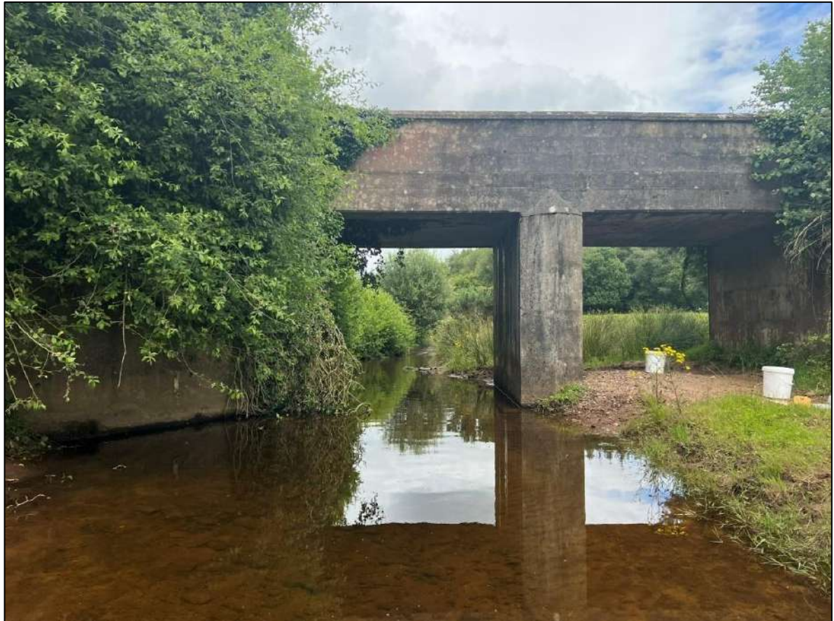
Plate 4-14. A representative photo of the bridge at survey site WF 8.
