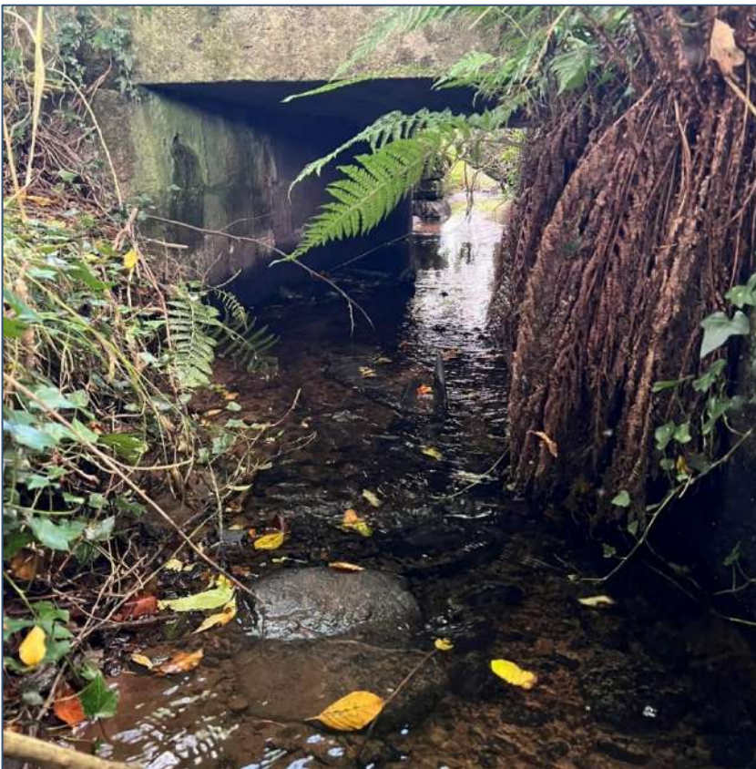
Plate 4-33. A representative image of the under-road culvert at survey location GC 6
