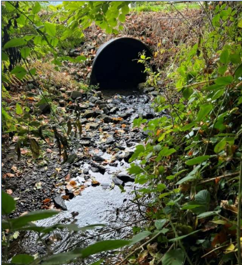
Plate 4-34. A representative image of the pipe culvert at survey location GC 6
