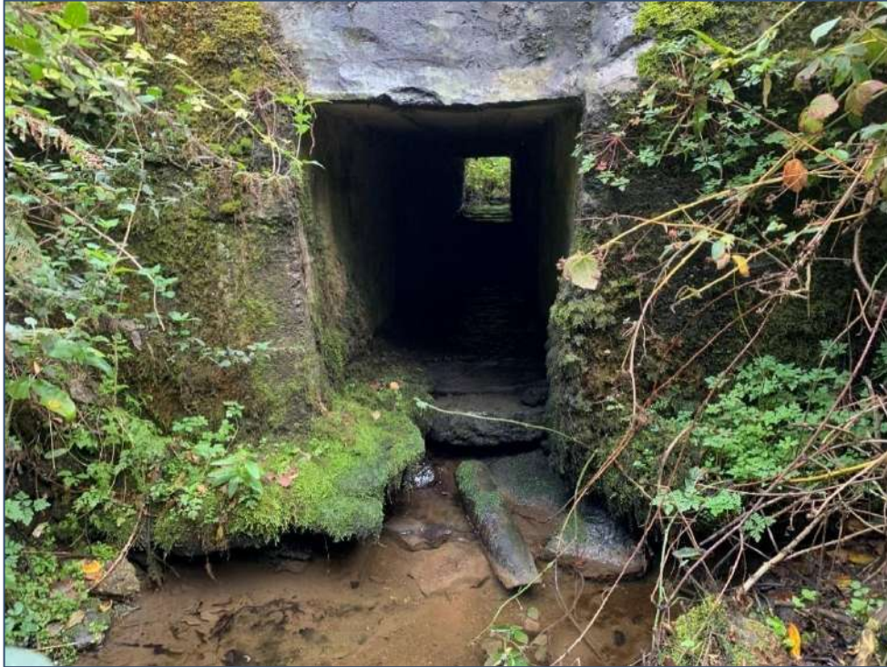
Plate 4-52. A representative image of the raised culvert at survey location GC 17
