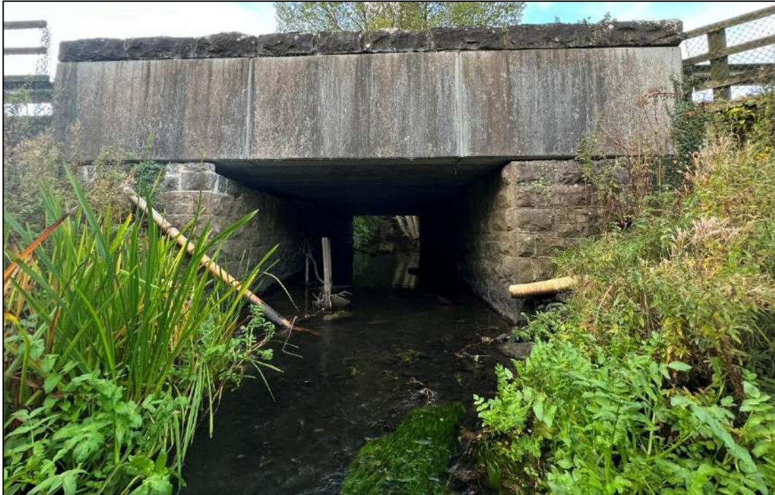
Plate 4-83. A representative image of the road bridge at survey location GC 35
