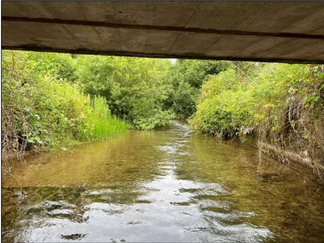
Plate 4-17. A representative photo of the upstream extent of Survey Site WF 10
