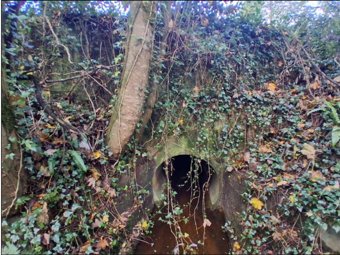
Plate 4-80. A representative image of the culvert at survey location GC 33
