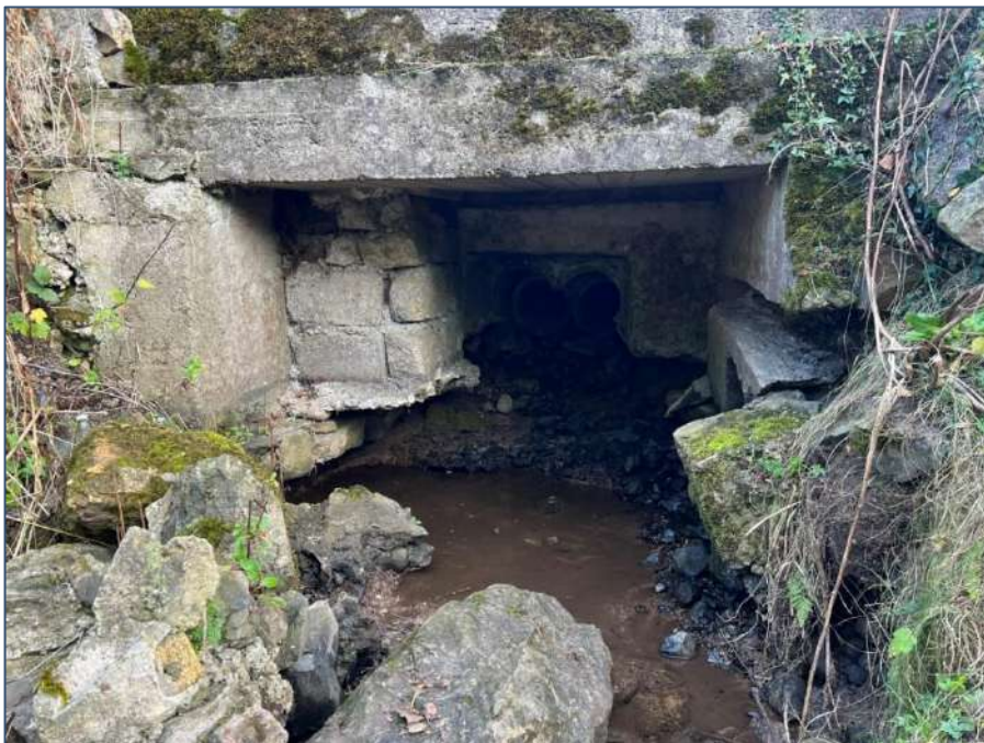
Plate 4-43. A representative image of the non-functional under-road culvert at survey location GC 11
