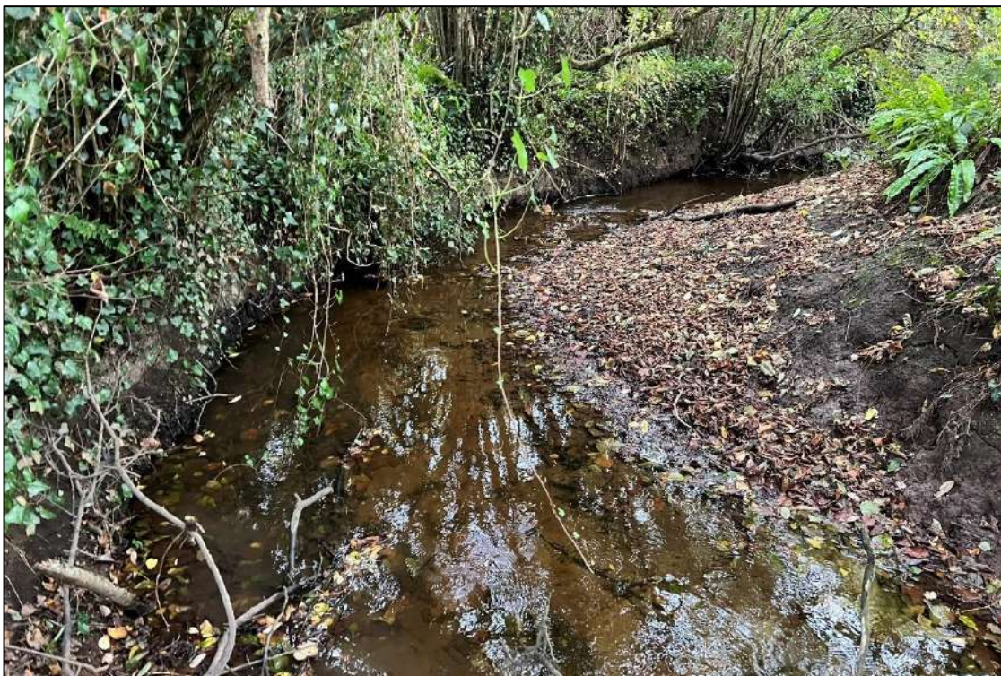
Plate 4-68. A representative image of the right-hand branch of the watercourse at survey location GC 27
