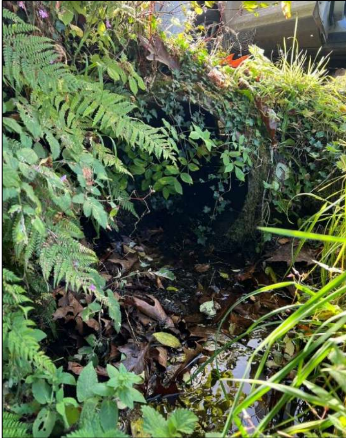
Plate 4-27. A representative image of the pipe culvert at survey location GC 2
