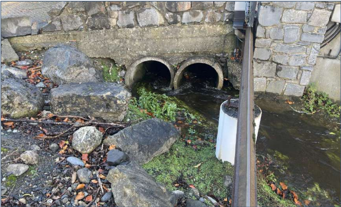
Plate 4-72. A representative image of the 2-pipe culvert at GC 29
