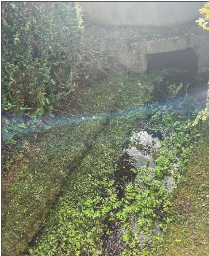
Plate 4-28. A representative image of the box culvert at survey location GC 2
